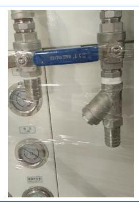
Open the side door of the chiller, and you will see the Y-shaped water filter of the equipment as shown
