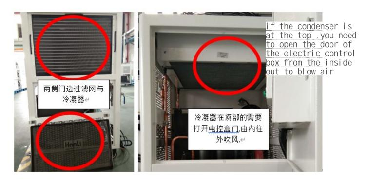
On both sides of the door side filter screen and condenser
